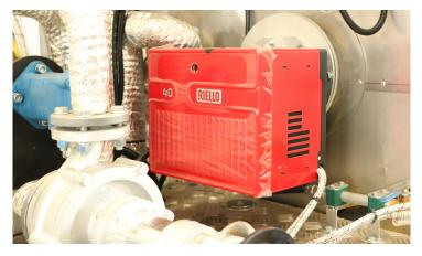
.Italy RELLIO diesel burner is applied.
